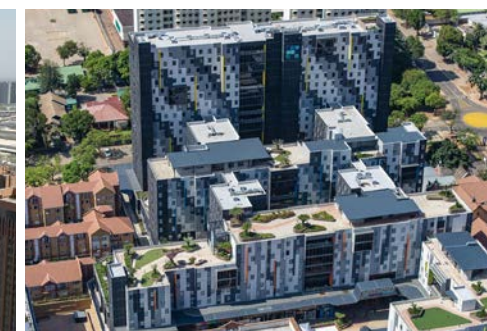
Hatfield Student Apartments, Pretoria, South Africa
